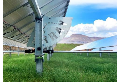
Racking mounted on piles
