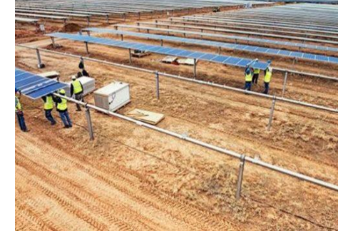
Panels installed on racking
