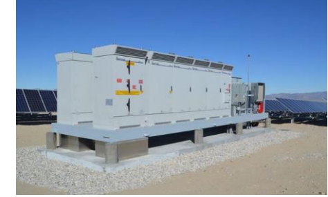
Inverter/transformer skid
